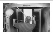
Low voltage cable has virtually no elasticity and should not be stretched by pulling. Pulling the low voltage cable can cause eventual failure.
